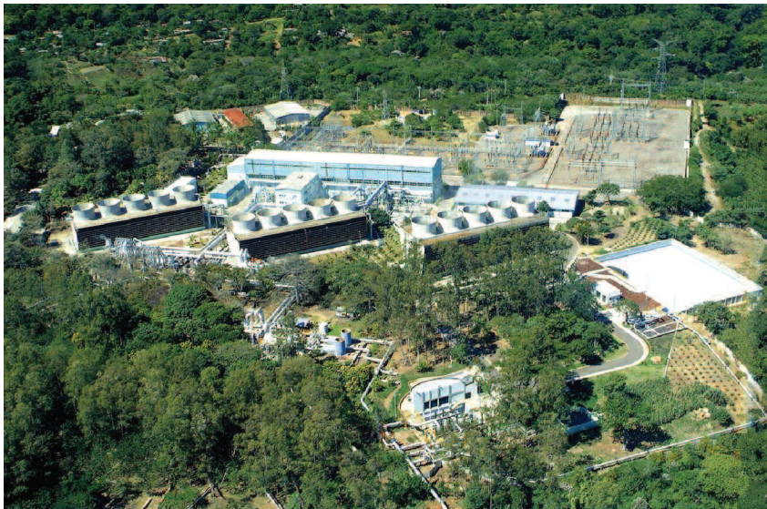
Figure 8.3 Ahuachapan geothermal facility after revegetation, circa 2005 (LaGeo, 2005).
